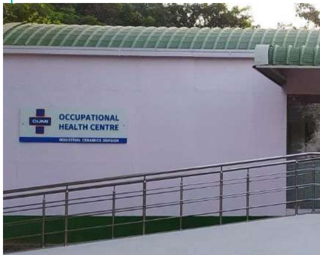
The Occupational Health Center at the Industrial Ceramics factory, Hosur, is constructed entirely using Coated Abrasives trim waste
